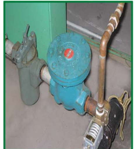
Condensate Assembly: Easily Accessible Basket Strainer/Steam Trap/Condensate Cooler
